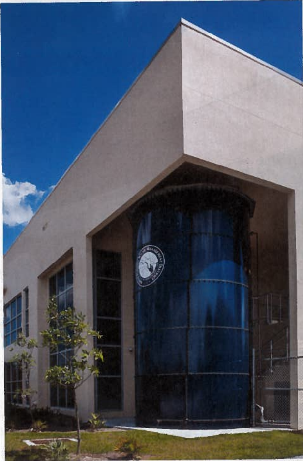
SFWMD regulates water use throughout South Florida, so the design team made the water cistern a focal point of the building design to showcase the district's commitment to water savings.
